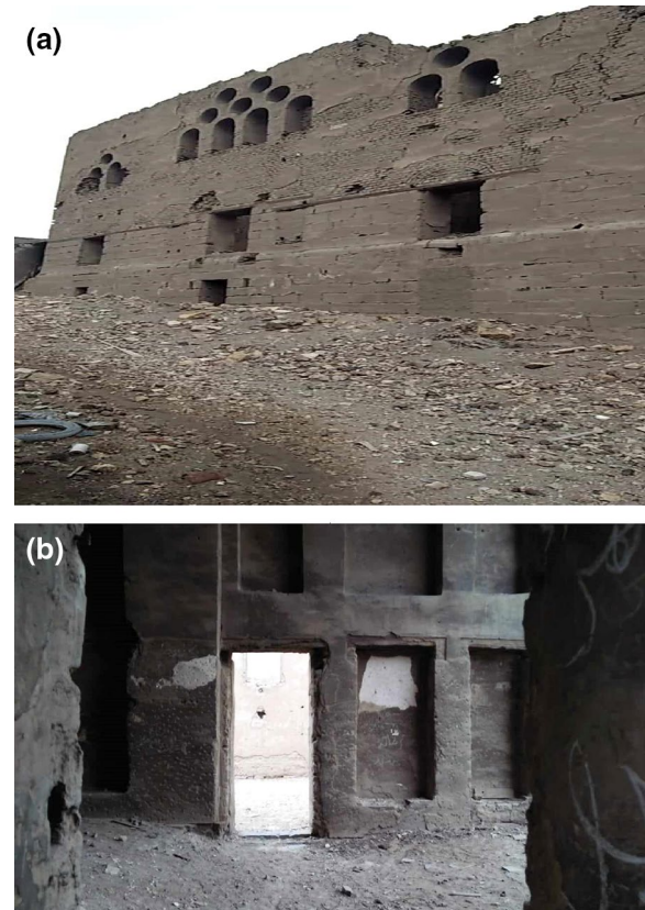
Fig. 4 a. In and out of plane deformations and distortions of the main façade are obvious. b. the state of preservation of the internal walls of the palace, the high raising of G.W.T and soiling of the stone walls is obvious
