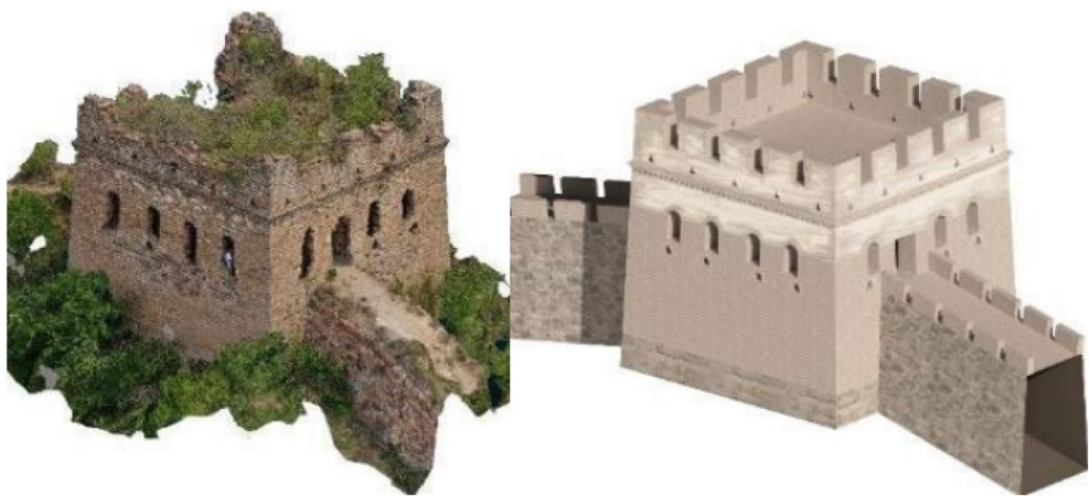
Fig. 11 Three-dimensional model of the current condition and restoration of the hollow watch tower
