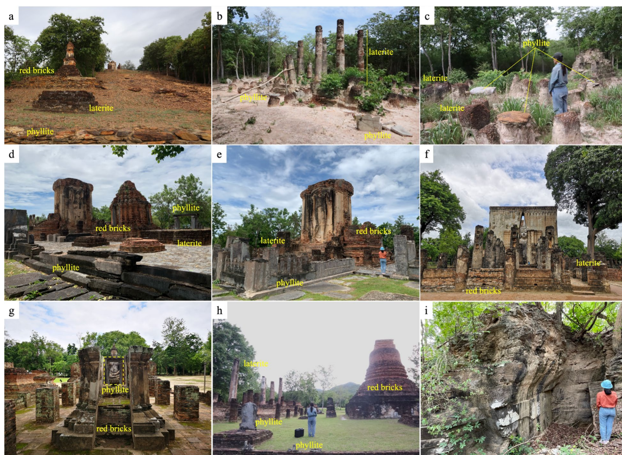
Fig. 3 Photographs of dimension stone used in the Sukhothai Historical Park and quarries of phyllite in Sukhothai Province. a Wat Saphan Hin Temple, b Wat Pa Daeng 2 Temple, c Wat Thap Sakae Temple, d, e Wat Chetuphon Temple, f, g Wat Sri Chum Temple, (h) Wat Mangkorn Temple, and (i) phyllite quarry at Wat Khao Noi Temple
