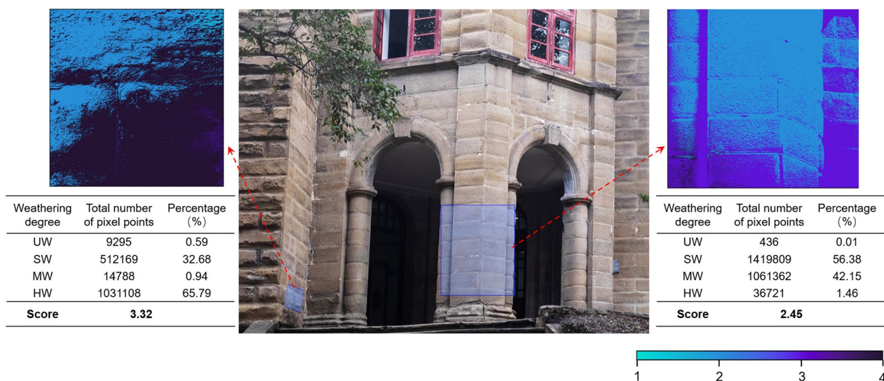
Fig. 15 Application of weathering assessment model in another sandstone building from the same stratum
