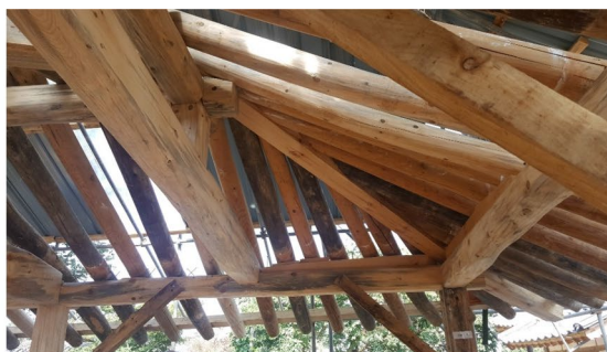
(b) Repaired wooden roof structure of the Gotaek
