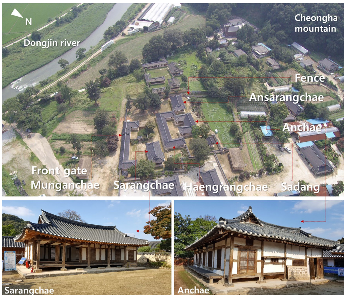
Fig. 1 Aerial photo and view of Korean traditional architectural heritage (Kim Myeong-KwanGotaek)
