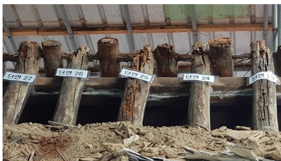
(a) Deteriorated wooden roof structure of the Gotaek
