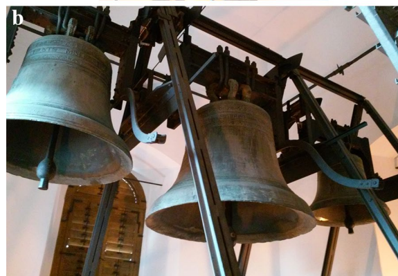
Fig. 2 a Bell "Urban", general view. b Bells and their supporting structure in the belfry of the parish church in Krosno, Poland
