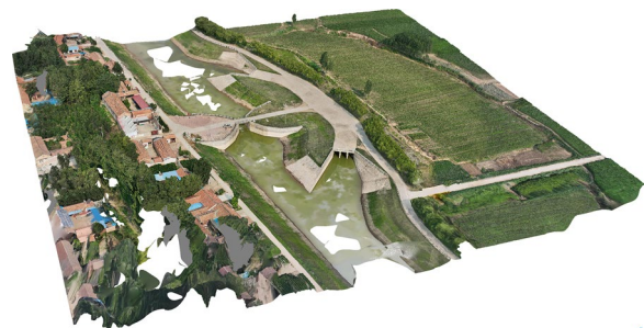
Fig. 7 Daiwan sluice gate
