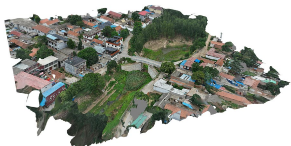
Fig. 11 Liulin sluice gate
