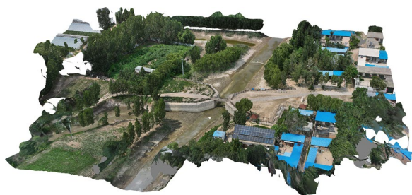
Fig. 8 A-cheng lower sluice gate
