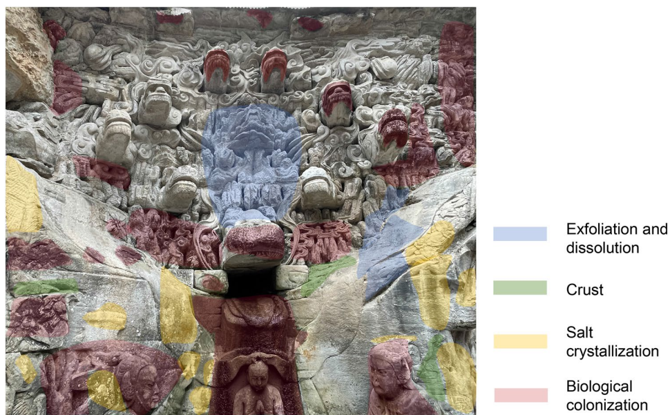
Fig. 3 Deterioration distribution map for rock carving of the Nine Dragons Bathing the Prince
