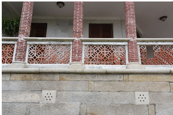
Fig. 6 The red-brick lattice railing is used to replace the red-brick bottle-shaped railing
