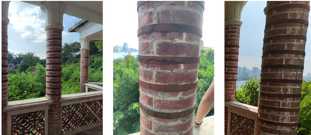
Fig. 5 The metal iron hoops are being used to support the columns
