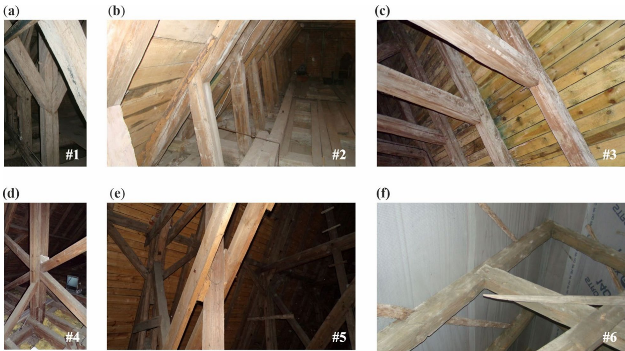
Fig. 6 Carpentry joints in church roof trusses: a Mitobądz (#1), b Pruszcz Gdański I (#2), c Kiezmark (#3), d Pruszcz Gdański II (#4), e Koźliny (#5), f Trutnowy (#6)
