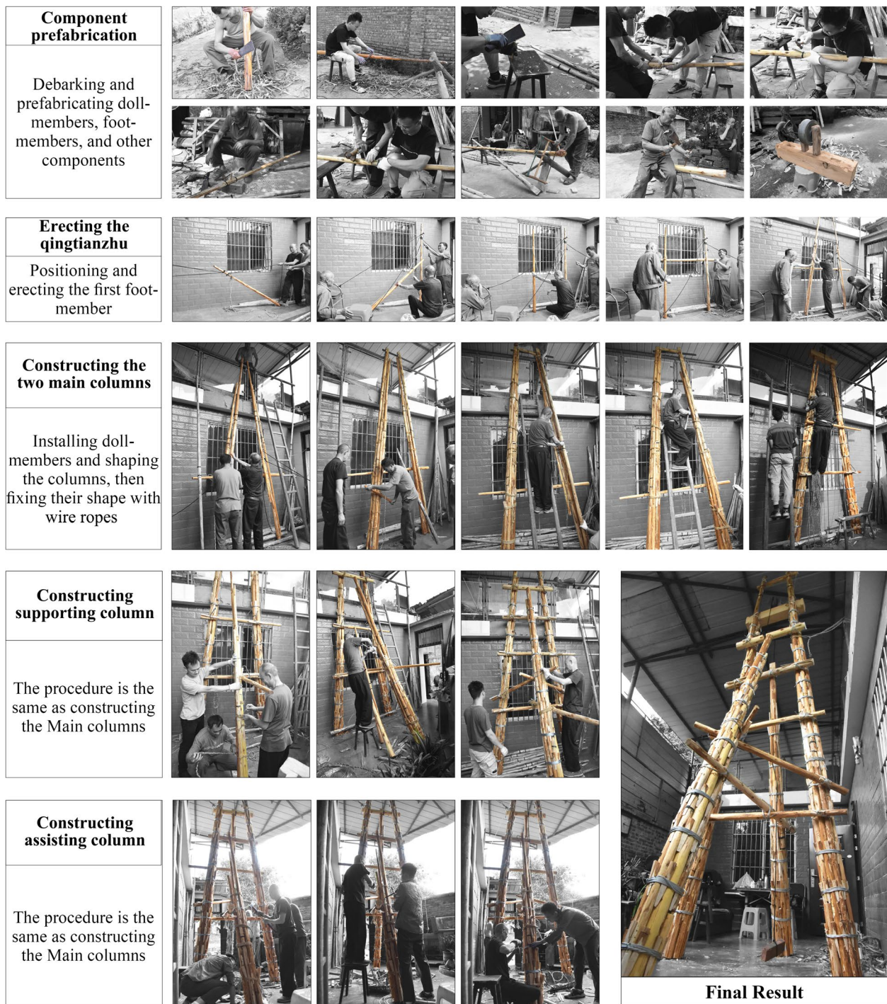
Fig. 7 Construction of a 5-m quadruple-legged Tianche model. Sources: the authors
