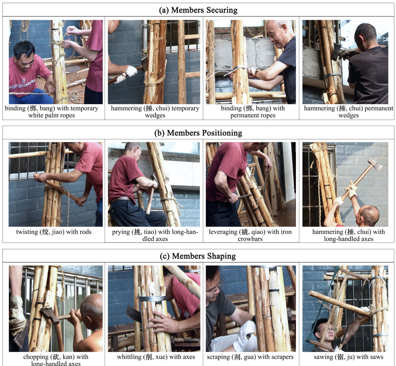
Fig. 6 Main construction techniques. Sources: the authors
