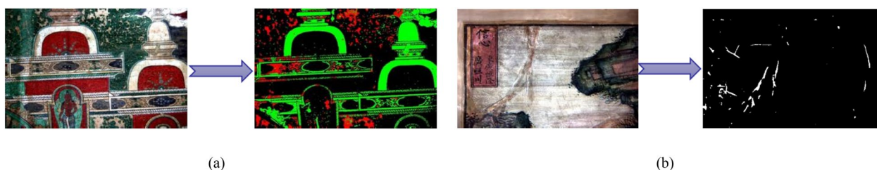
Fig. 5 Extraction results of architectural heritage surface diseases: a the results obtained by the extraction method of shedding diseases based on the combination of spectrum and shape; b scratch extraction results based on improved U-Net
