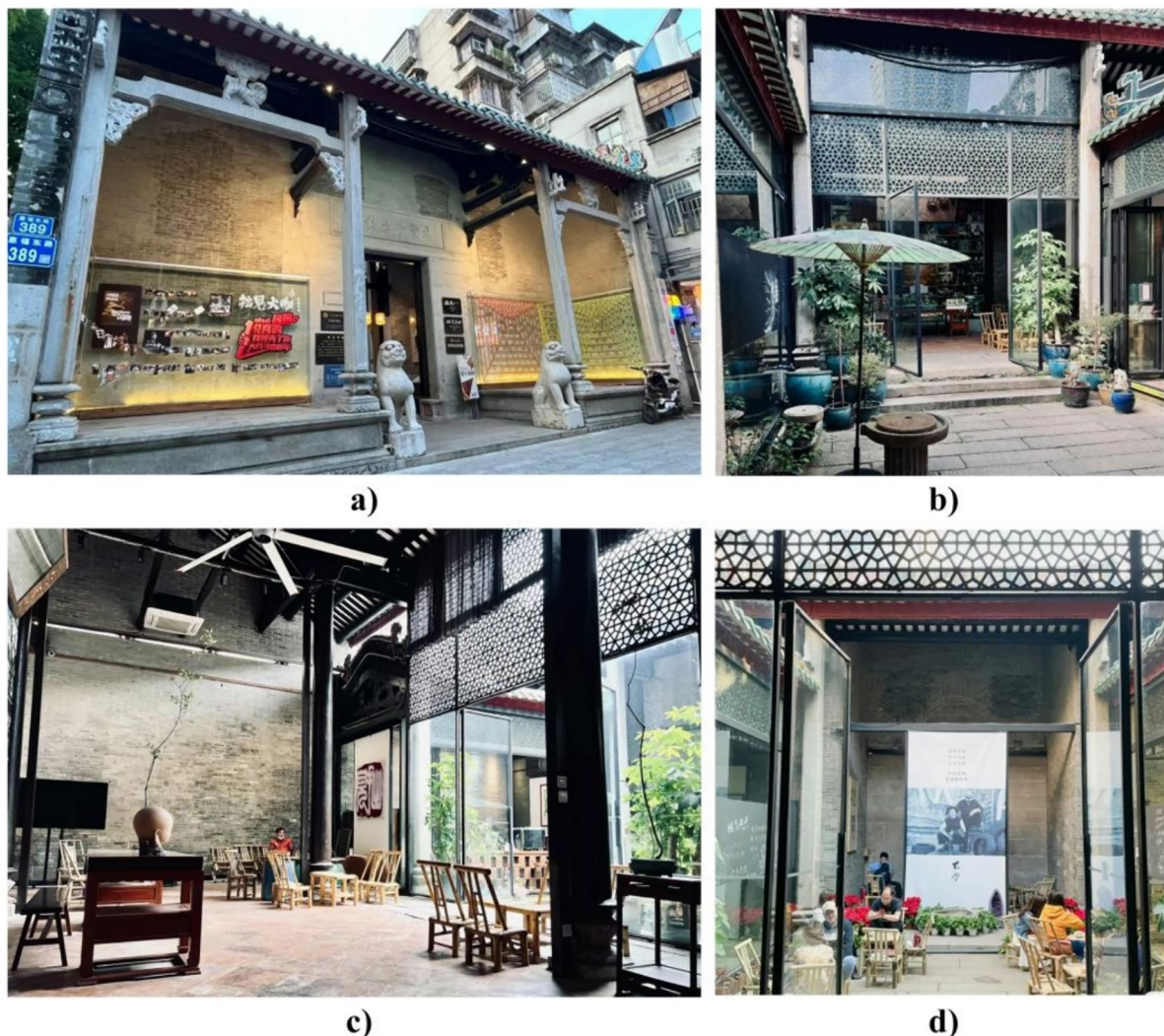
Fig.3 Qingyun Academy's indoor renovation and utilization involves enclosing the courtyard with glass curtain walls (Source: Own illustration)
