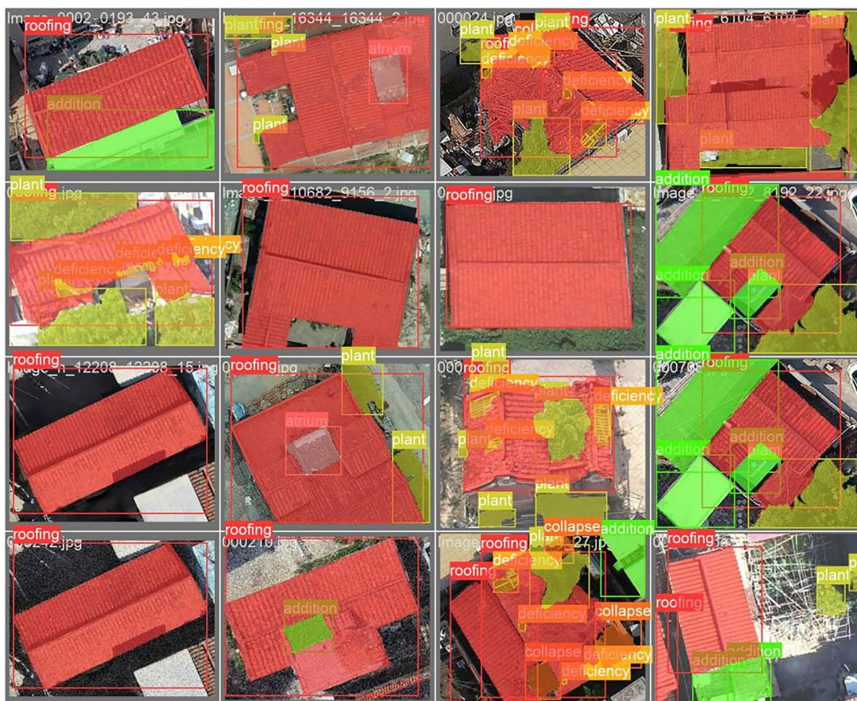
Fig. 13 Roof damage inspection results
