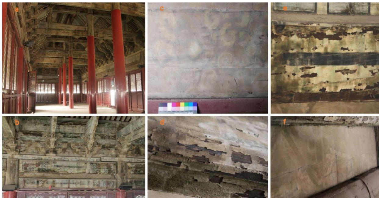
Fig. 2 Typical diseases on color paintings of the archery tower at West Gate (a: overall preservation condition; b: local condition; c: faded; d: cracked; e: fallen off; f: covered by dust.)
