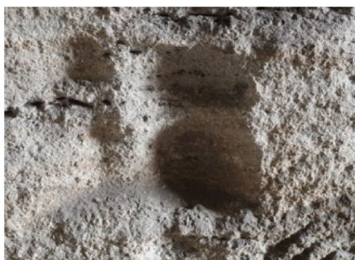
(a) Powdery weathering
