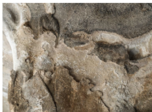
(b) Sheet-like weathering
