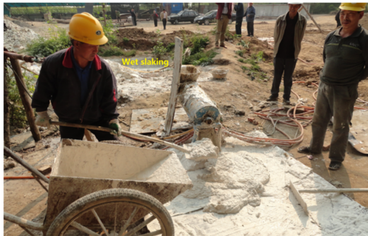
Figure 3 Wet slaking and preparation of lime with hemp fibers during restoration works in southern Shanxi 2012.
