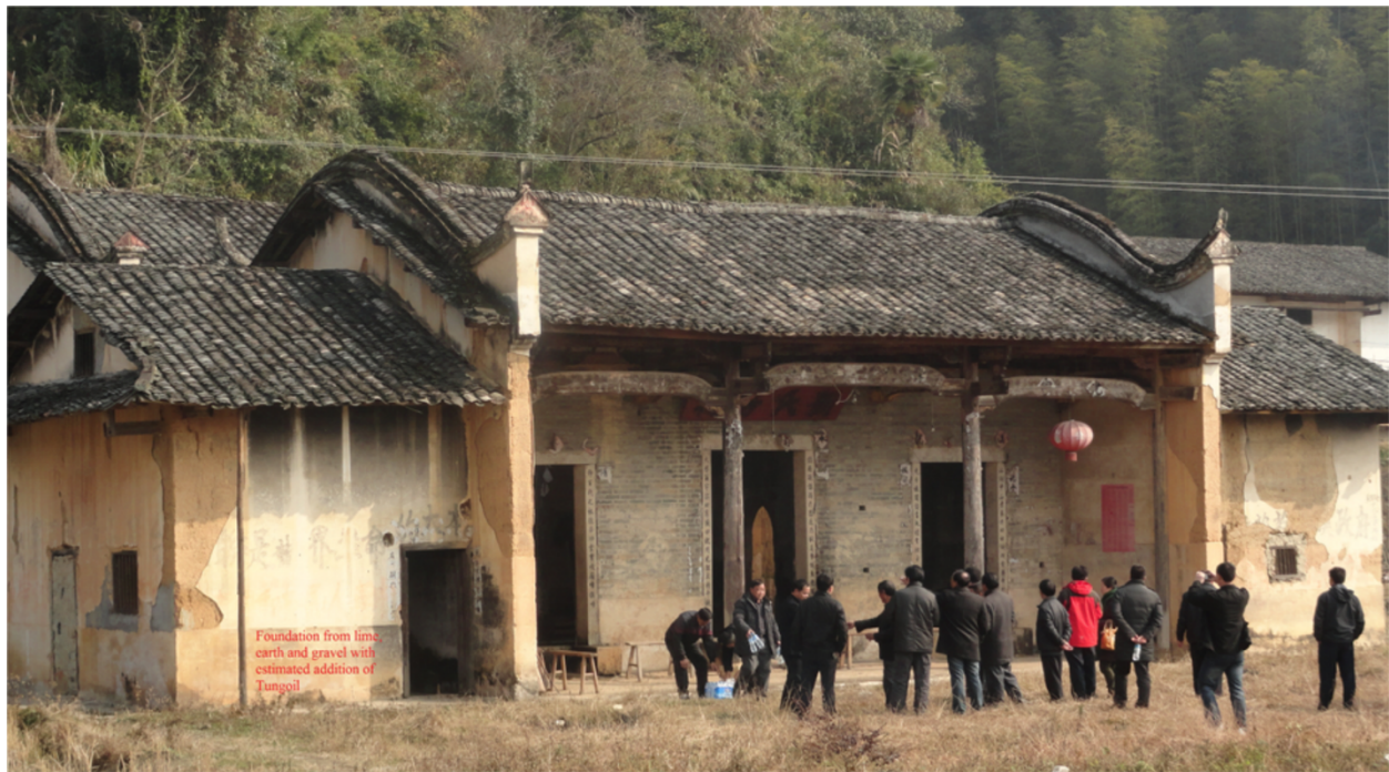
Figure 5 Traditional earthen-timber architecture built in 1824 with foundation from lime, earth and gravel with estimated addition of Tungoil in Jiangxi Province.
