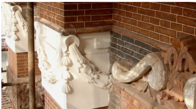
Figure 8 Strawed dispersed lime to restore marble imitated ornaments in Xuhui High School Shanghai (built in 1850).
