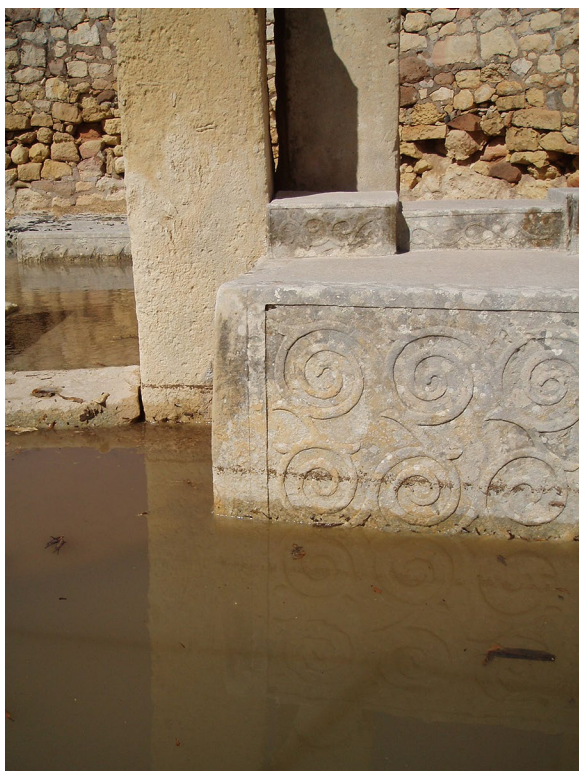
Fig. 7 Persistent flooding within the Tarxien Temples after heavy rains regularly reached 30 cm in depth
