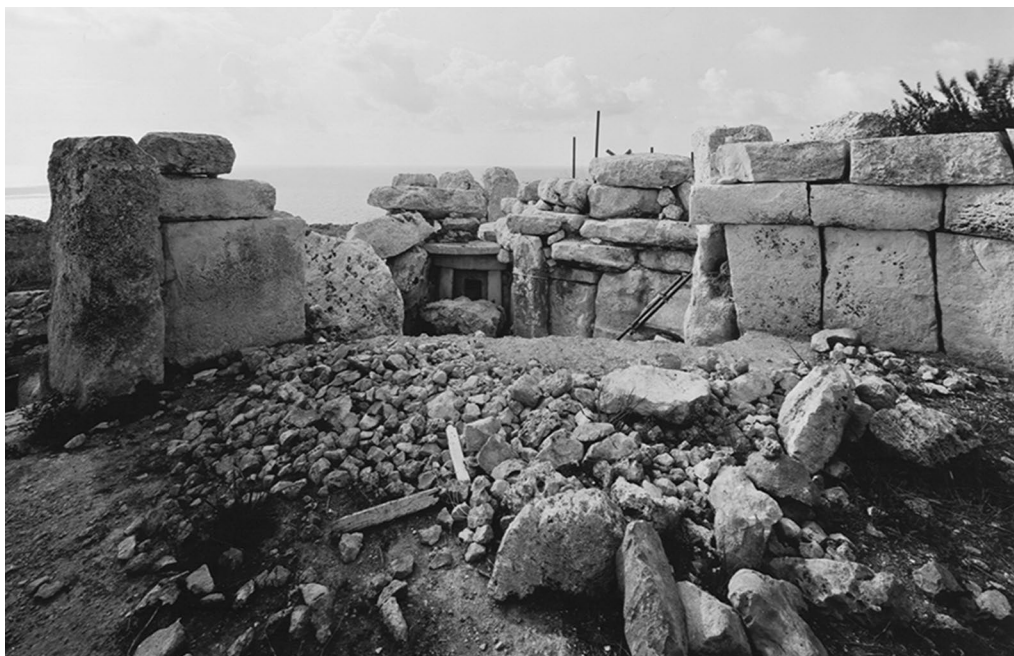
Fig. 5 Collapse of part of Mnajdra Temples, 1996, following heavy rainfalls with loss of structural stability
