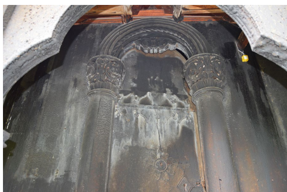
Fig. 2 The southern door and portal of Hopperstad Stave Church, partly covered by a white layer. A data logger, to monitor the temperature and RH, is visible in the upper right part of the picture
