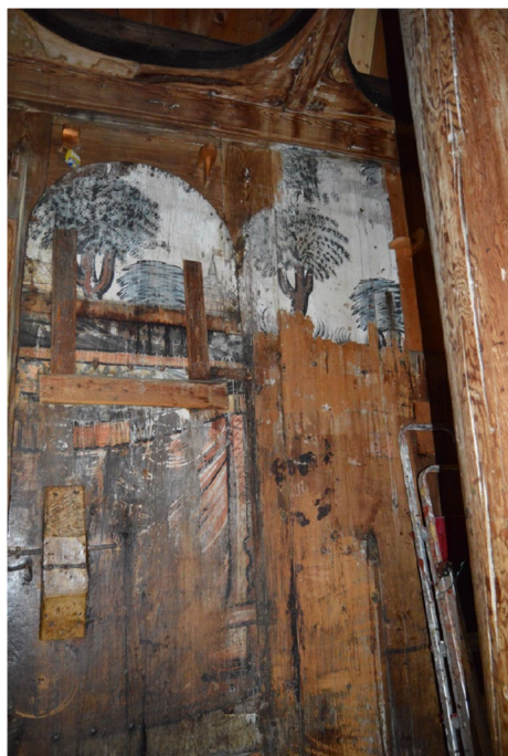
Fig. 11 Glue paint on the interior of the southern door and wall
