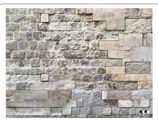
**Fig. 1** Reigate Stone masonry at the Bell Tower, Tower of London, showing high level of variability. Majority of masonry is in Reigate Stone, with range of block colours and sizes, and decay patterns and rates. Second and third course are replaced with other lithologies (except central stones); approximately 15 stones on right of picture also replacement lithologies. Boundary between Reigate and other stone marked by black border
